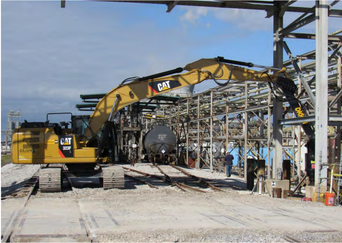
Fig. 8. Limited Access Helical Pile Installation (Courtesy of Cajun Deep Foundations, LLC)
