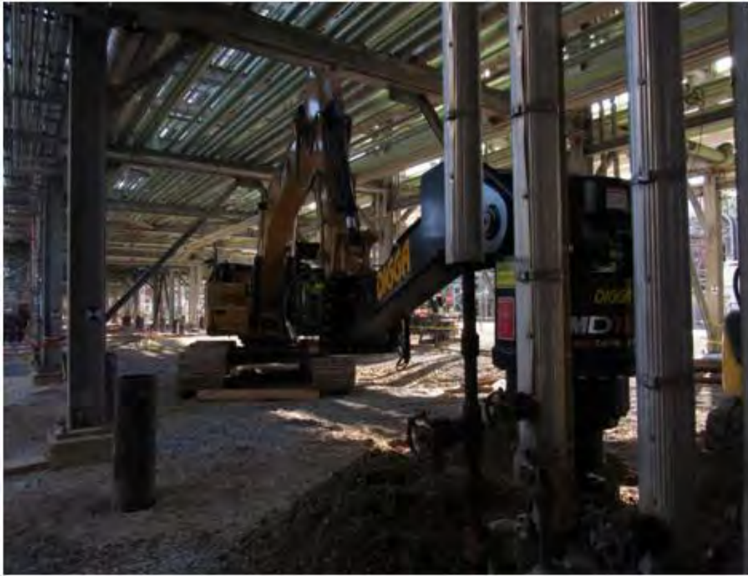
Fig. 10. Confined Area Helical Pile Installation (Courtesy of Cajun Deep Foundations, LLC)
