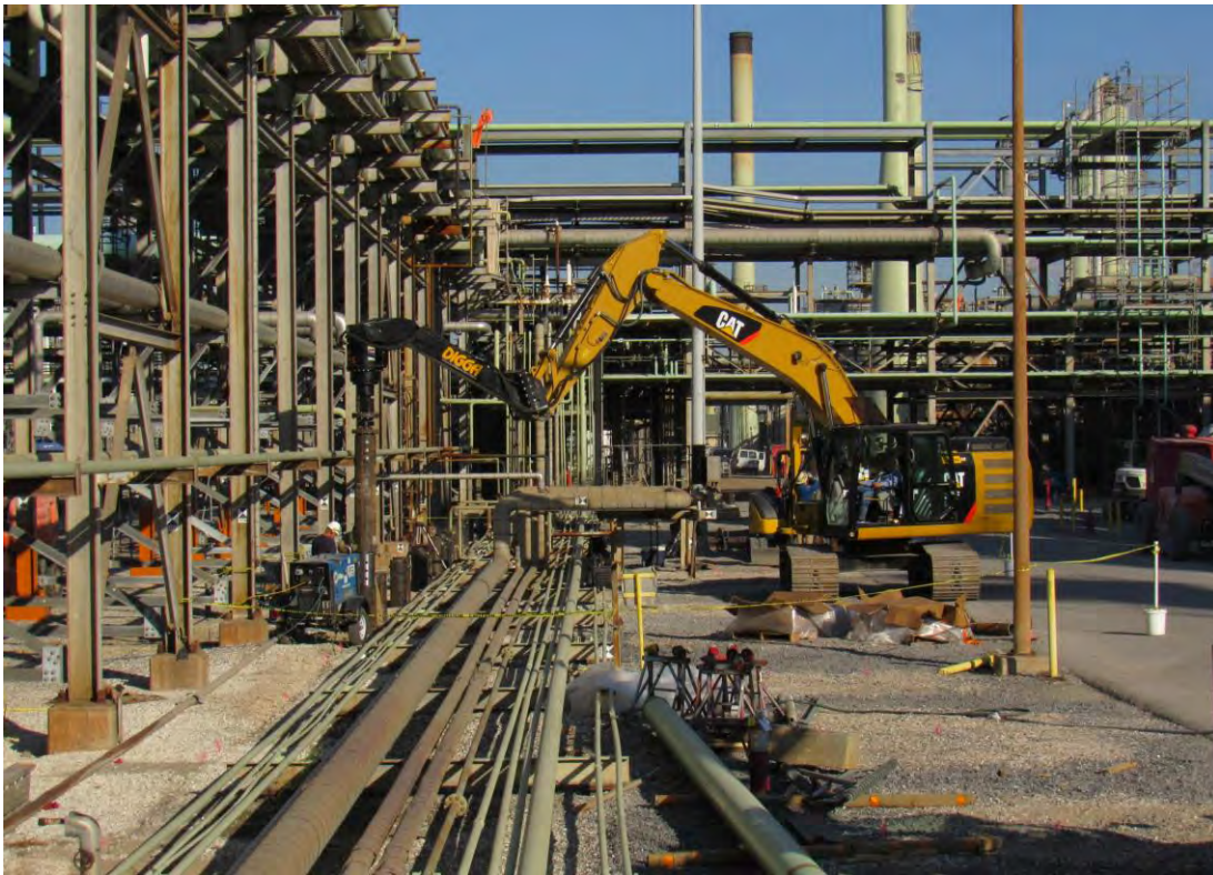
Fig. 9. Cross Equipment Helical Pile Installation (Courtesy of Cajun Deep Foundations, LLC)
