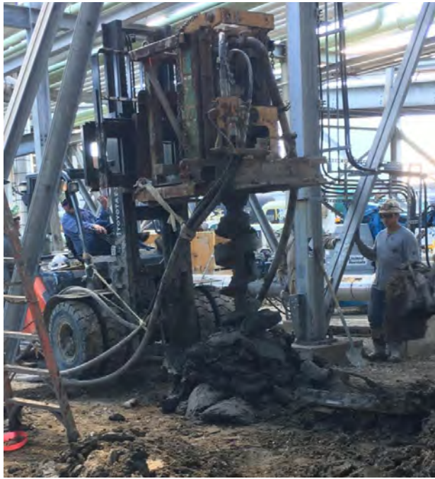
Fig. 3. Low Overhead Auger Cast Pile Installation (Courtesy of Fluor Corporation)
